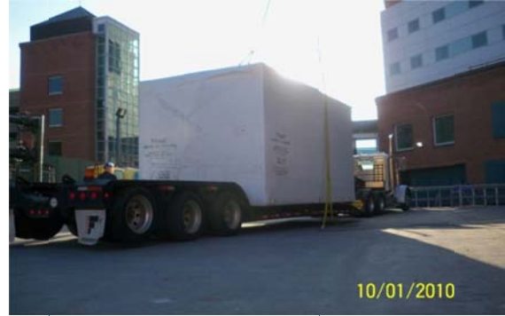
Fig. 3 shows a new air plenum arriving on site.
