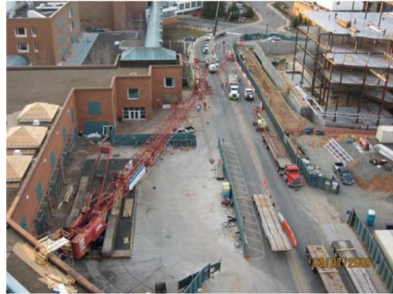
Fig. 7 shows the erection of a 888 crane
